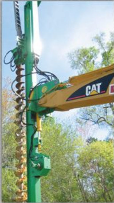
Set up for pile predrill
