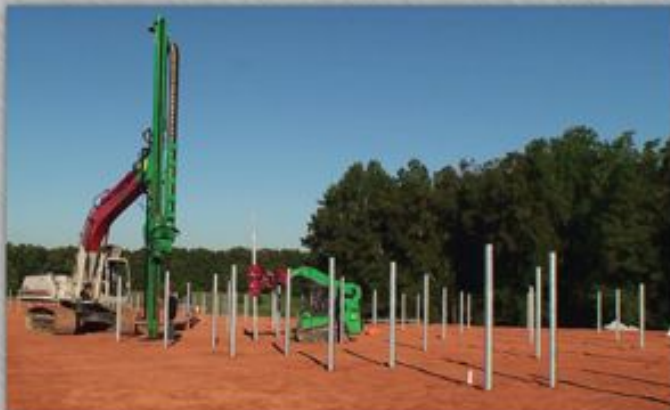
Solar field foundations
